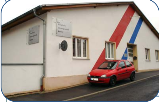
The new building in Kamenz.
